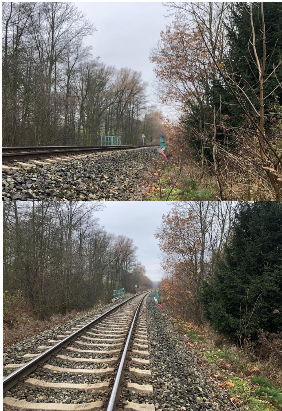
Nová deformace GPK v km 26,0
